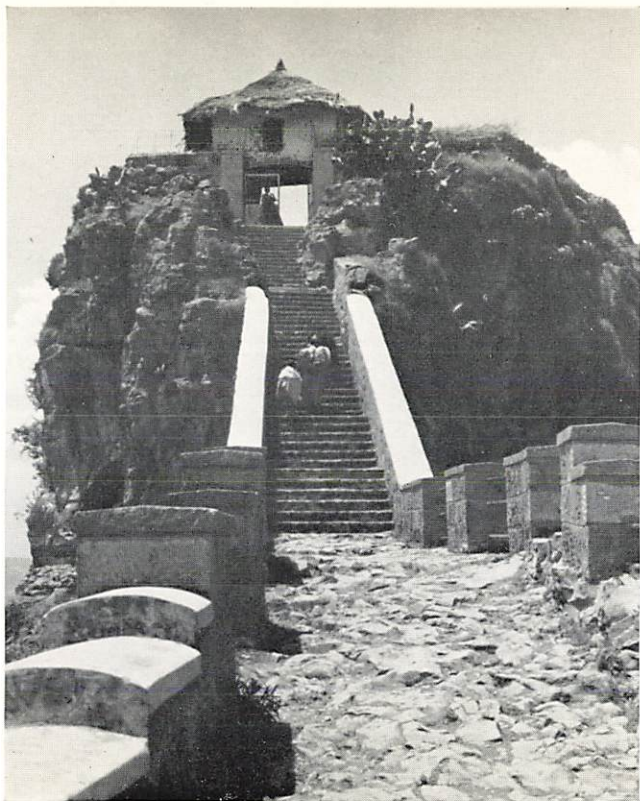
The only gate to the mountain top
